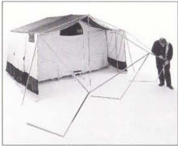
5. Connect the three roof poles to the front 'A' frame. NOTE: The lower leg section can be left 'broken' at this point to give a lower working height.
