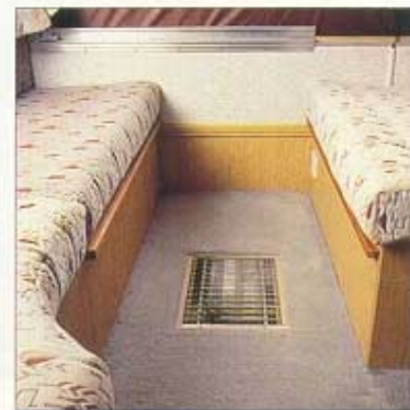
Under floor heater
