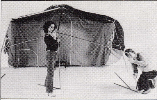
21. Add side cabin roof poles and legs leaving bottom of front support legs broken.
