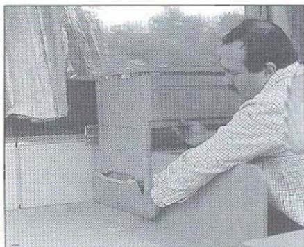
**14.** Now lift the kitchen unit at the left hand side and secure at the correct height by seating on top of the hinged flap. Unclip the waste hose beneath the sink and locate in the opening in the base unit.
