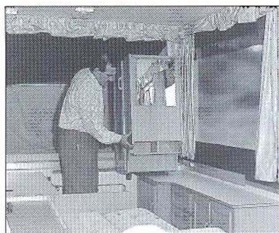
12. When vertical - slide the wardrobe across and into position on top of the cupboard units.
