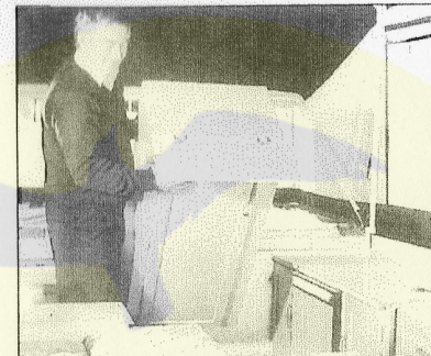
11. Lift over wardrobe and slide onto locker top. Locate four bed stop pins into holes in bed runner slides.
