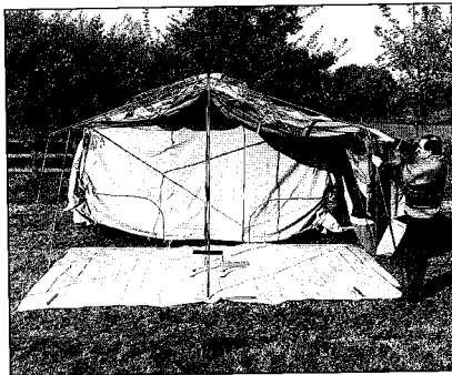
7. Connect the three roof poles to the front 'A' frame then add the two centre legs. Pull forward the extension canvas from the cabin roof.
