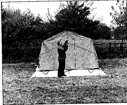
5. A & B. - Connect the centre roof pole to the front 'A' frame. Repeat for the two side roof poles.
