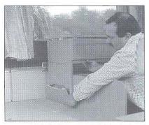
14. Now lift the kitchen unit at the left hand side and secure at the correct height by seating on top of the hinged flap. Unclip the waste hose beneath the sink and locate in the opening in the base unit.
