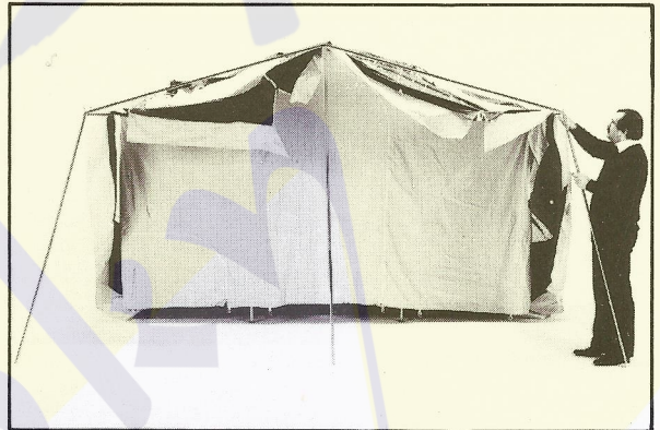
6 Pull canvas forward from roof of cabin section.
