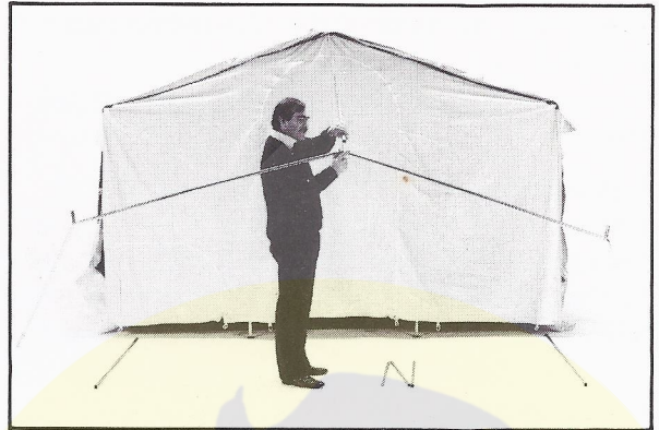
3 Connect centre roof pole to front extension 'A' frame.
